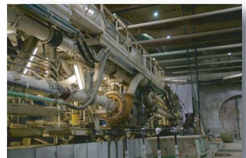
TBM "Leonie", City Tunnel Leipzig
